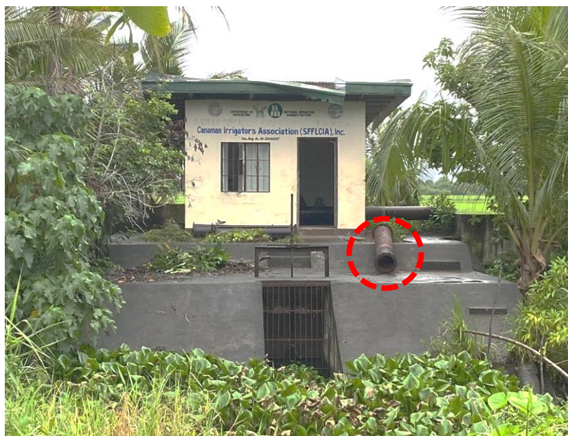
Figure 2. Detached irrigation facility established by NIA in Mangayawan, Canaman
